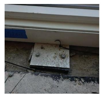
Figure 8 — Window Wall façade frame fasted via HAC-TU and Selfdrilling screws
