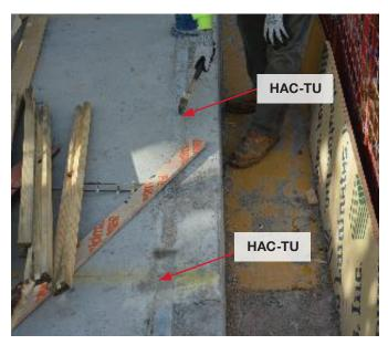
Figure 2 — HAC-TU cast-in concrete
