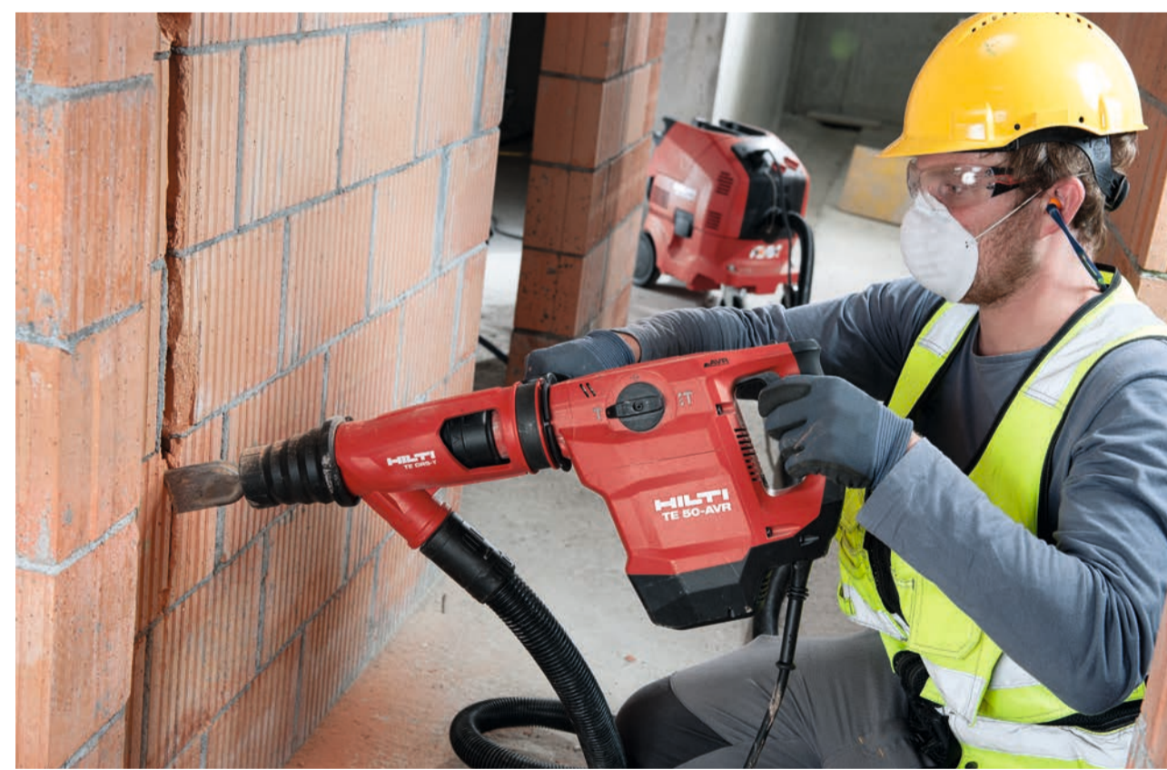
TE 50-AVR: medium range anchor hole drilling, light chiseling
