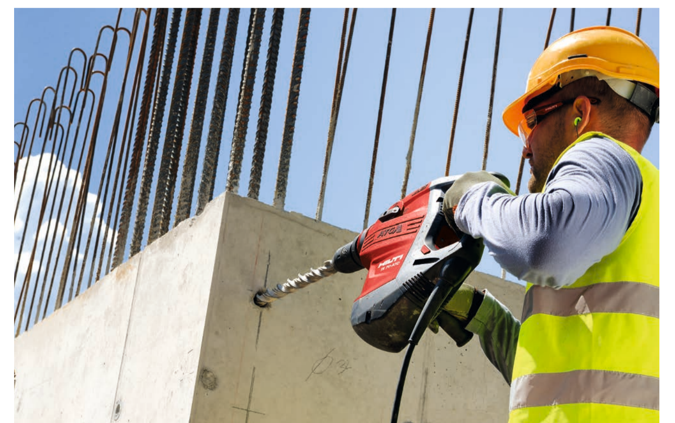
TE 70-ATC-AVR: Rebar doweling, large anchor hole drilling
