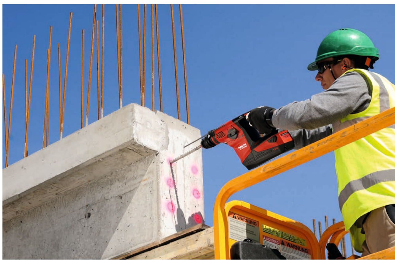
TE 30-A36 Cordless: limited access area drilling, light chipping
