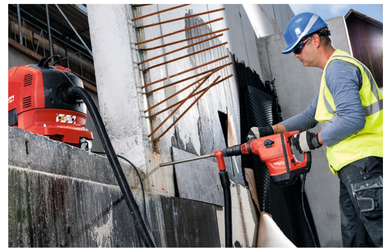
TE 60-ATC-AVR: Rebar drilling, medium-duty demolition work
