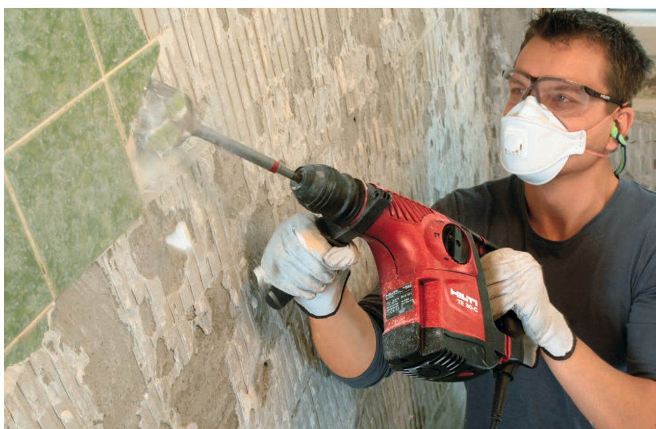
TE 30-C-AVR: light chipping, small range anchor hole drilling
