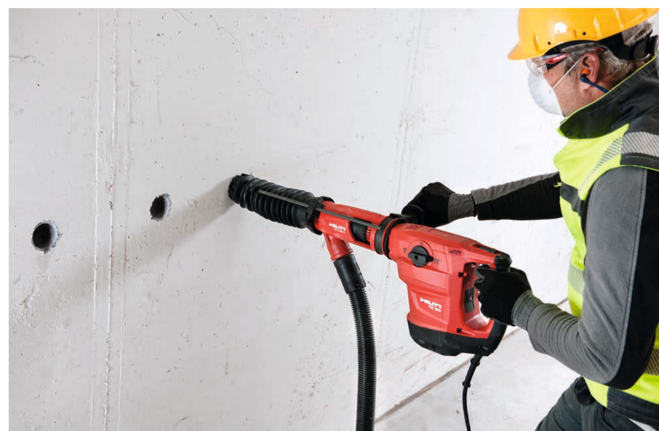
TE 60-AVR: Pipe penetration core drilling in concrete with DRS solution
