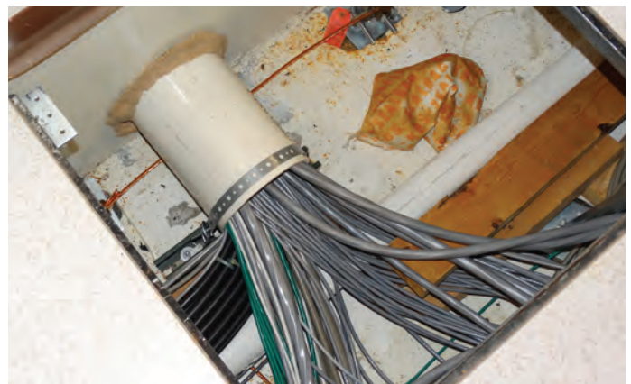
FIGURE 1: Firestop bag initially inside of sleeve was not replaced after cabling additions or modifications.
