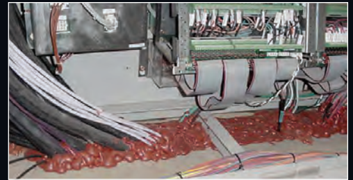
FIGURE 3: Intumescent (heat-expanding) firestop foam can provide nearly perfect L ratings as it flows and hardens between cables.
