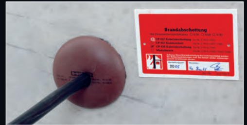
FIGURE 5: Penetration firestopped with intumescent flexible foam plug.
