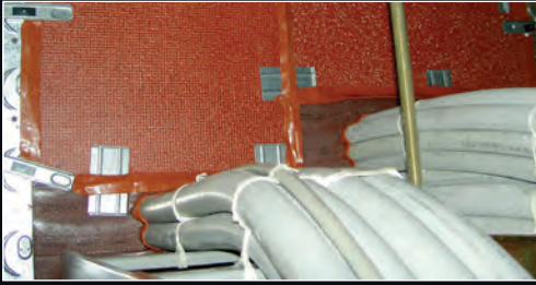
FIGURE 7: Service penetration opening with firestop board.
