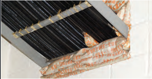
FIGURE 8: Firestop bags (note that mandatory retaining wire mesh on each side of the wall is missing).
