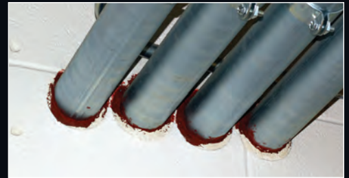
FIGURE 2: Conduit penetrations permanently firestopped with caulk-based system.
