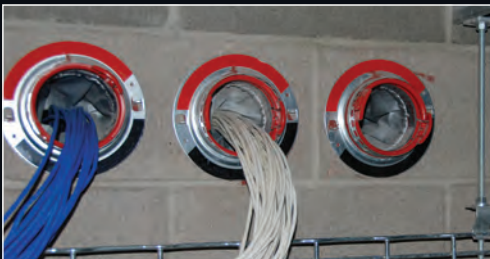
FIGURE 10: Preinstalled firestop sleeves.
