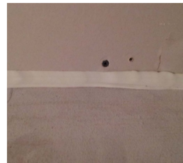
Bottom-of-Wall Joints
